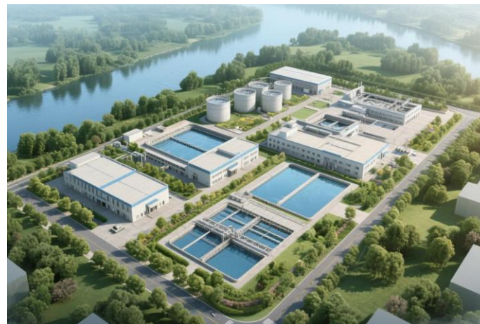
Municipal water plant renovation
