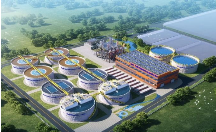
12,000 m 3 /d Printing & Dyeing Wastewater Zero Discharge Project in Morocco
