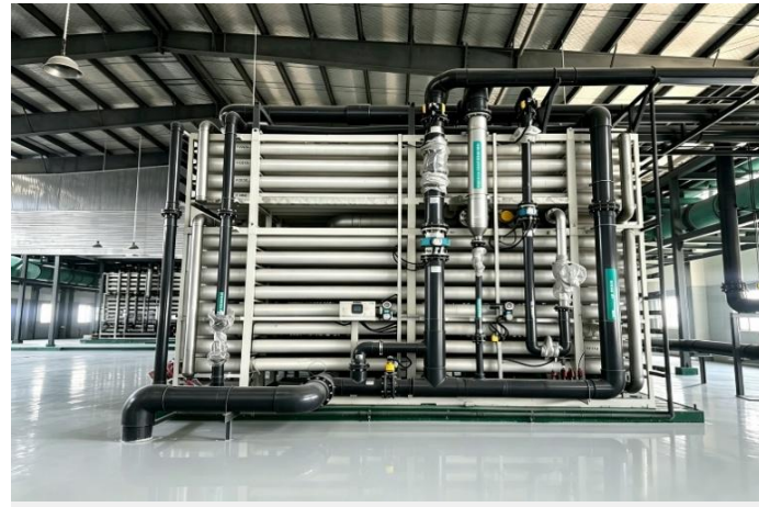
28,800 m 3 /d Steel Wastewater Reuse Project in Jiangxi
