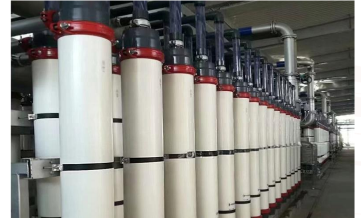
20,000 m 3 /d Municipal Water Supply Project in North China
