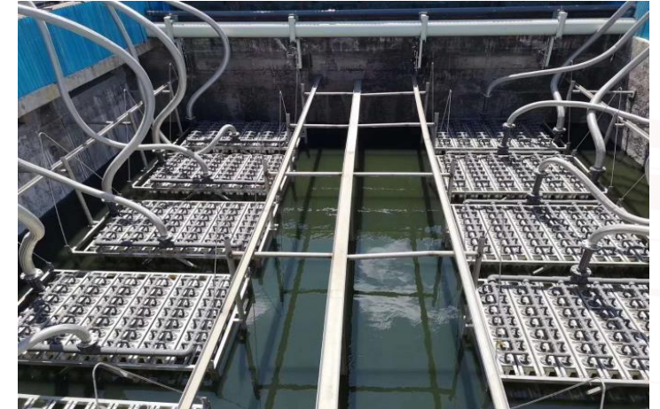
4,800 m 3 /d Coal-to-methanol Wastewater Treatment Project in Yunnan
