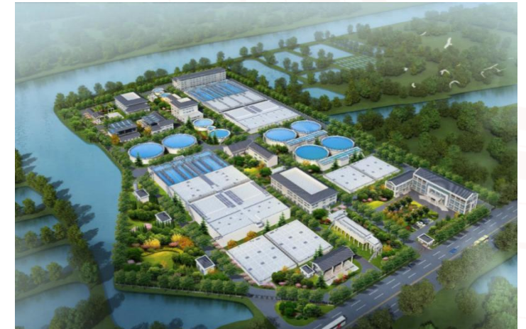
25,000 m 3 /d Industrial Wastewater Treatment and Reuse Project in Zhejiang
