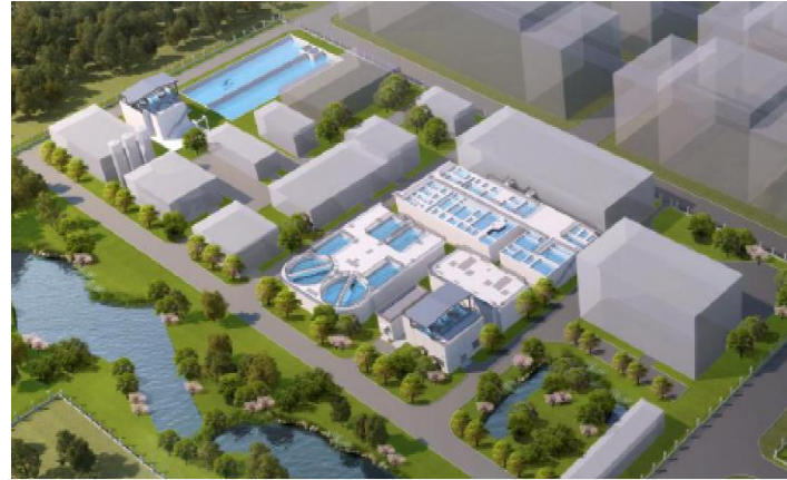
1,200 m 3 /d Electroplating Wastewater Reuse Project in Anhui
