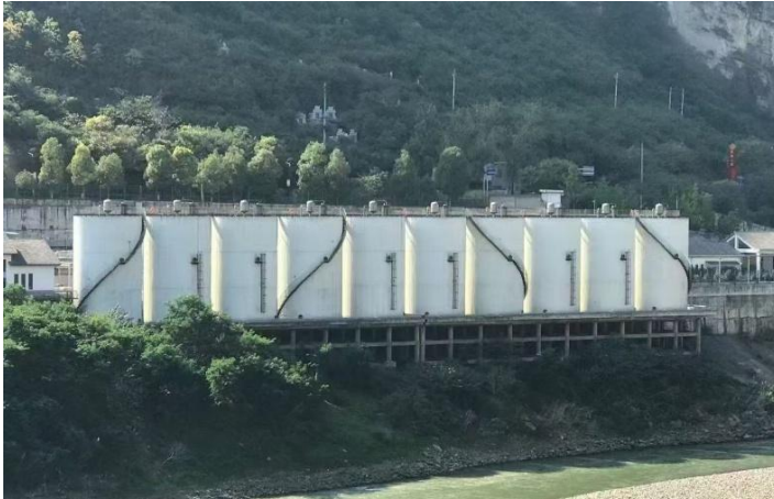
5,000 m 3 /d Baijiu Wastewater Treatment Project in Sichuan
