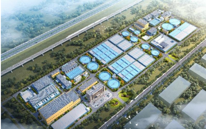
100,000 m 3 /d Papermaking Wastewater Treatment and Reuse Project in Anhui
