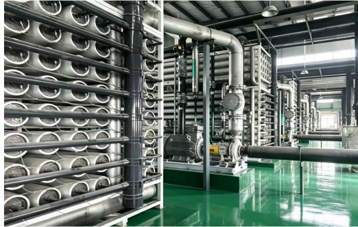
7,000 m 3 /d Industrial Park Wastewater Treatment Project in Kendari
