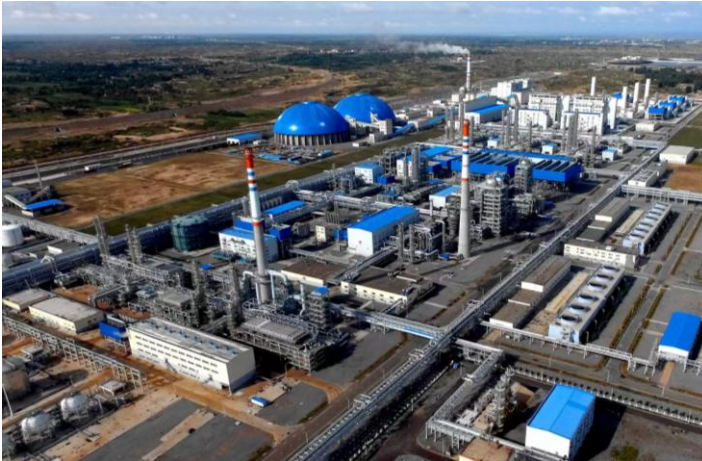
29,000 m 3 /d Coal Chemical Wastewater Treatment & Reuse Project in Inner Mongolia
