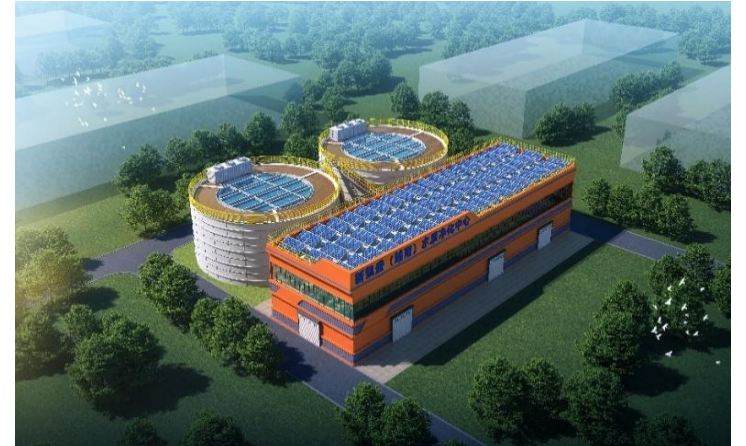
6,000 m 3 /d Printing & Dyeing Wastewater Reuse Project in Vietnam
