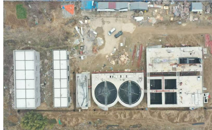
1,000 m 3 /d Dairy Wastewater Treatment Project in Jiangsu
