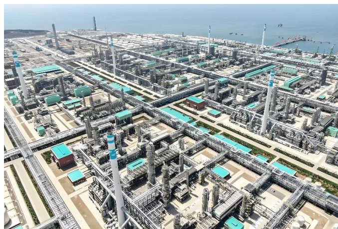
Emergency water supply for the factory
