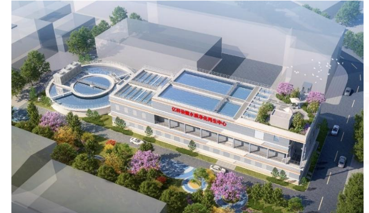
10,000 m 3 /d Printing & Dyeing Wastewater Treatment and Reuse Project in Fujian
