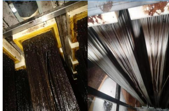
1,000 m 3 /d Semi-coke Wastewater Treatment Project in Shaanxi
