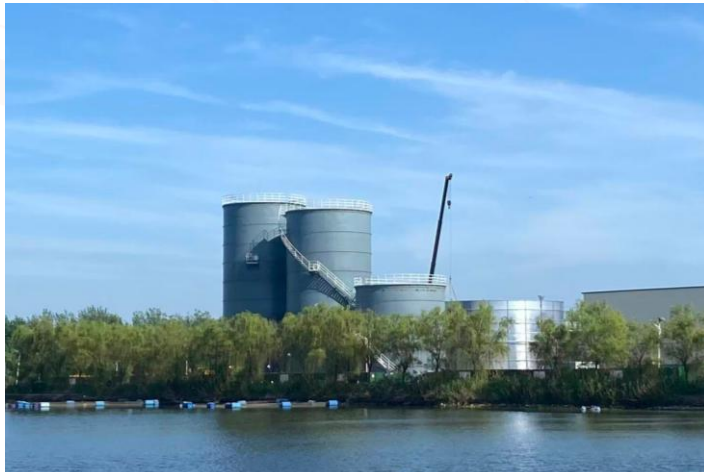
1,000 m 3 /d Food Wastewater Treatment Project in Anhui
