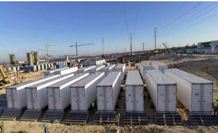
20,000 m 3 /d Seawater Desalination Project in Morocco
