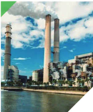
FLue gas desulfurization
